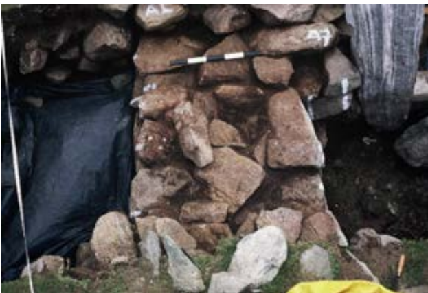
Illus 12.70 Gaps at the top of 769 [Film 1981.12.35]
